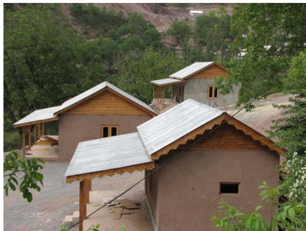
Temporary classrooms nearing completion
