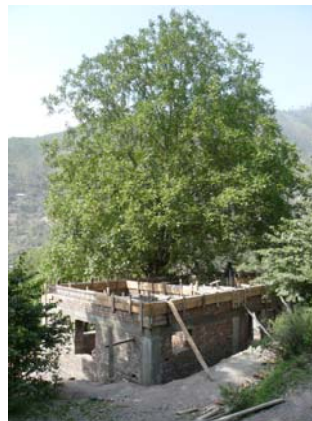
A teacher residence under construction. Teachers will be accommodated on campus
