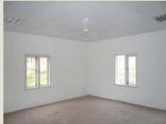
One of the temporary classrooms recently completed
