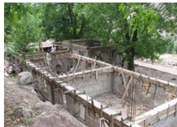
Work in progress on the first academic block
